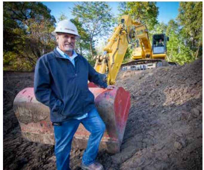
Geddis Paving & Excavating president, Steve Oliver, onsite in Toledo, Ohio with a Komatsu PC290LCi excavator.
