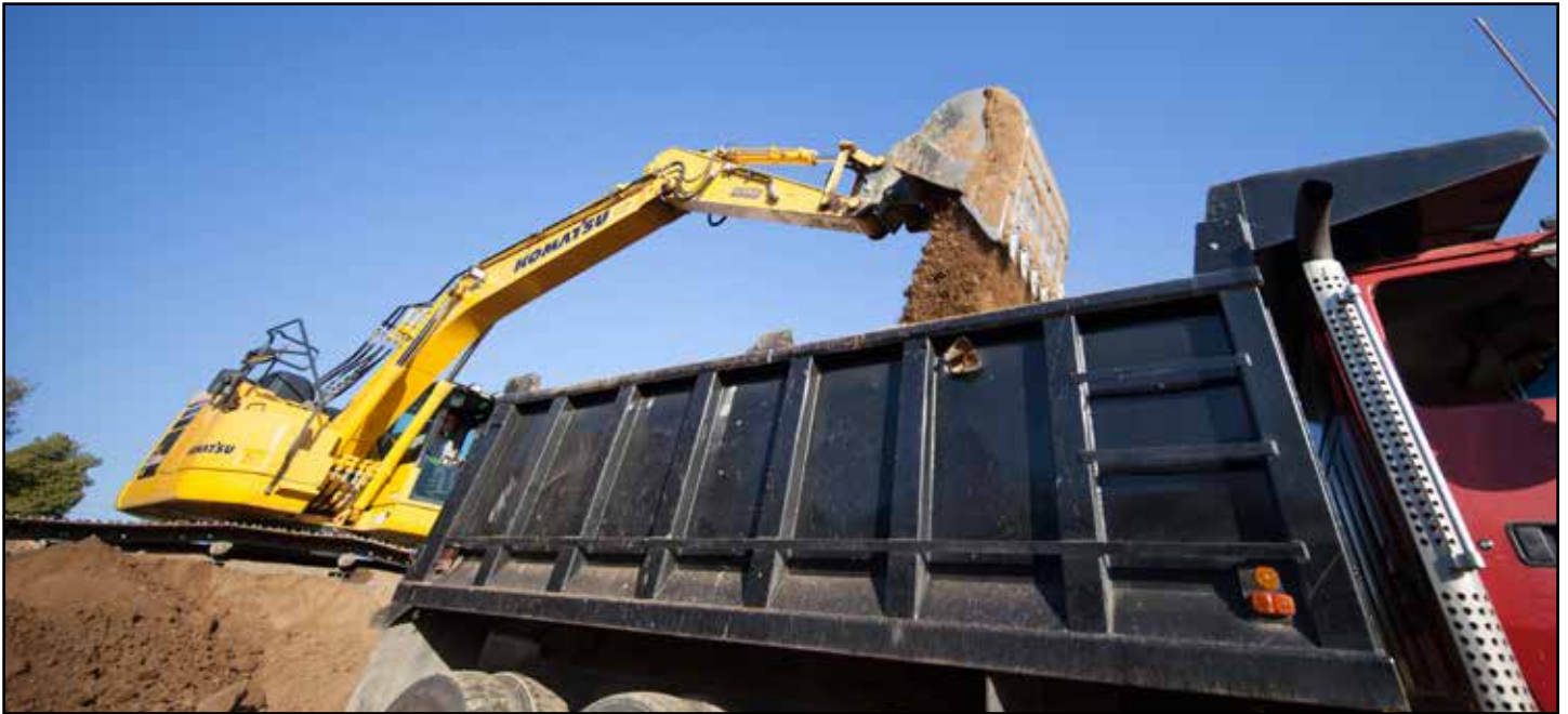
A T.C. Holzen Komatsu PC238USLC moves some of the 5,900 cy of dirt on a $677,000, Casey's General Store retail petroleum project located in Carlisle, Ohio.
