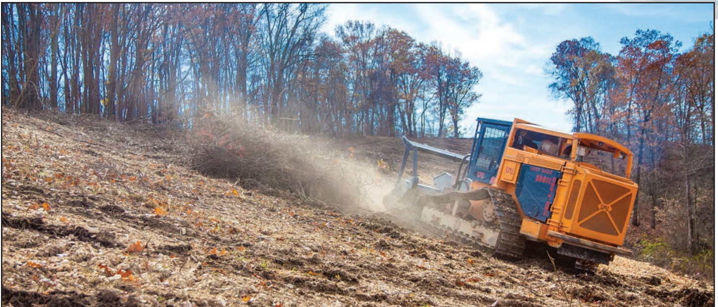
North Suburban Tree's CMI C450 mulcher—pictured clearing land around Range Resources' John Elliott 11826 well in Canonsburg, PA—needs to be "tough, well-engineered and safe", as Blum described, to handle unforgiving environments that can encompass 1,000 acres.
